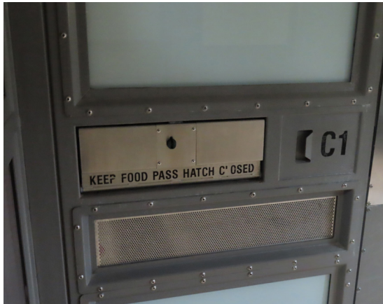
Photo 4 - Close-up of mesh panel in cell door in Murgon watch-house.
