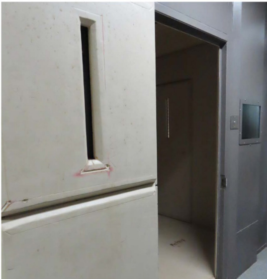
Photo 23 - Padded detention cell at Murgon.
