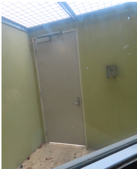
Photo 17 – The disused exercise yard at the Murgon watch-house.
