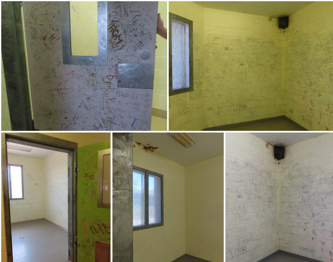
Photos 16–20: Separation rooms
